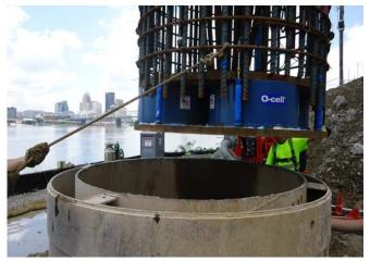
O-cell placement at the end of reinforcement cage
