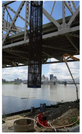
Reinforcement cage installation with O-cells
